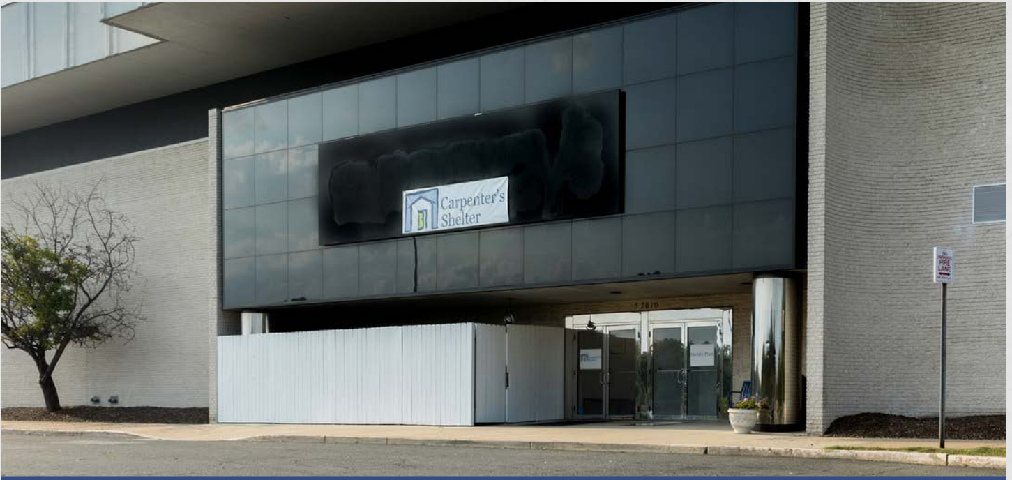
CARPENTER'S SHELTER'S TEMPORARY LOCATION INSIDE THE FORMER MACY'S AT LANDMARK MALL
